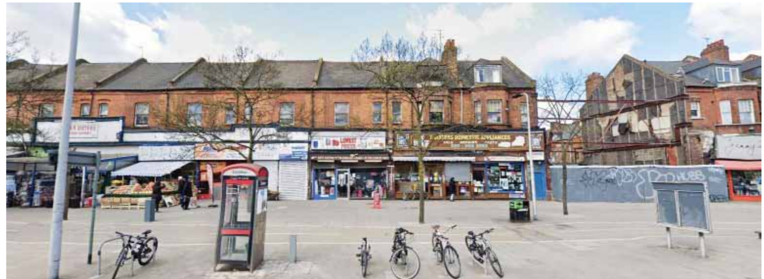
16. View of 245-249 High Road with the gap in the terrace visible (right, the application site) Tottenham High Road
