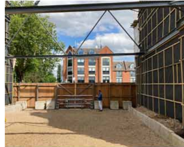
45. Existing view towards High Road from within site
