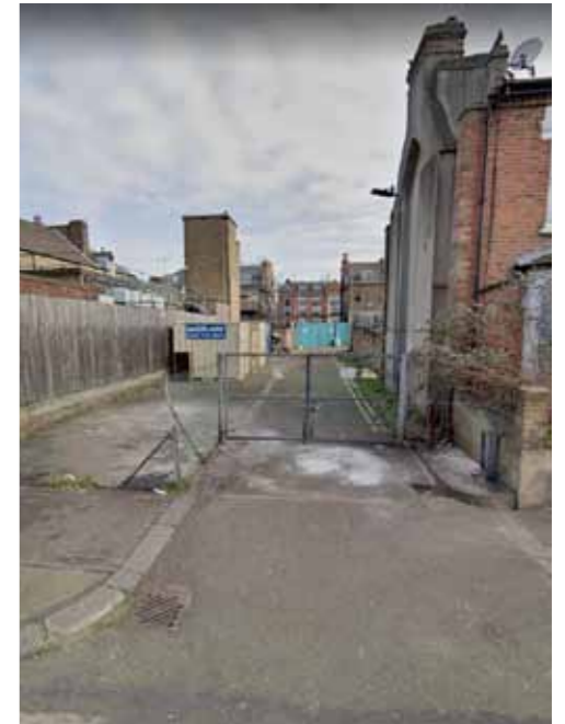
15. Rear Access Road Exit Gate Suffield Road
