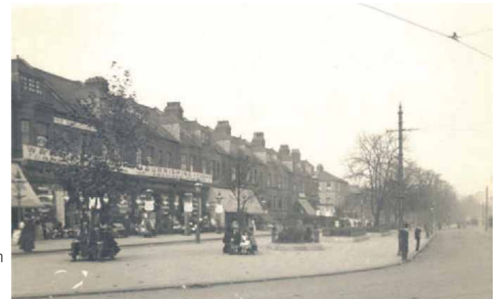
34. Archive Image looking North-Westward along the High Road with the terrace 227-259 (left)
