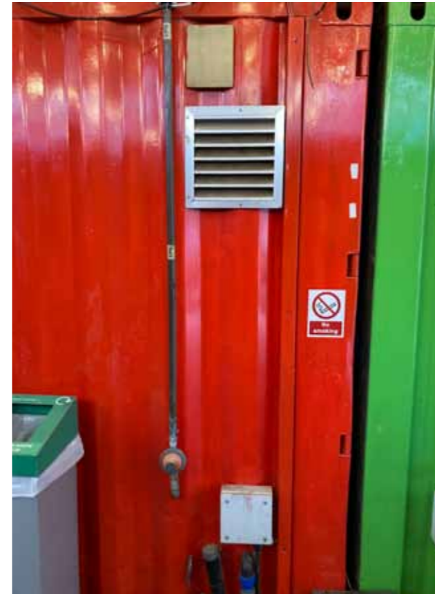
40. Examples of 10ft converted shipping containers with simple services and extract ventilation
