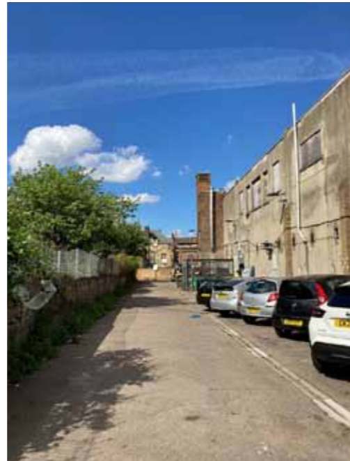
13. View Along Rear Access Road
