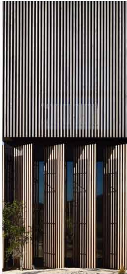
Hit and miss timber cladding
