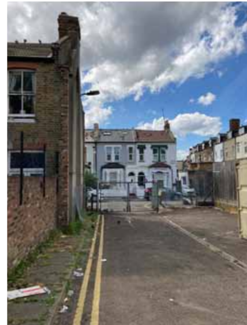
14. Rear Access Road Exit Gate Rear Access Road
