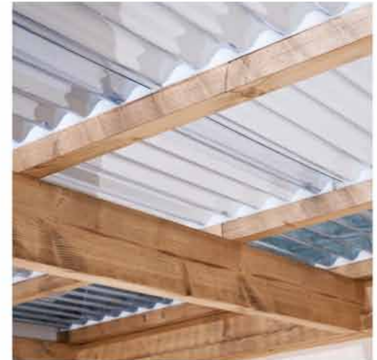
Polycarbonate and timber pergola
