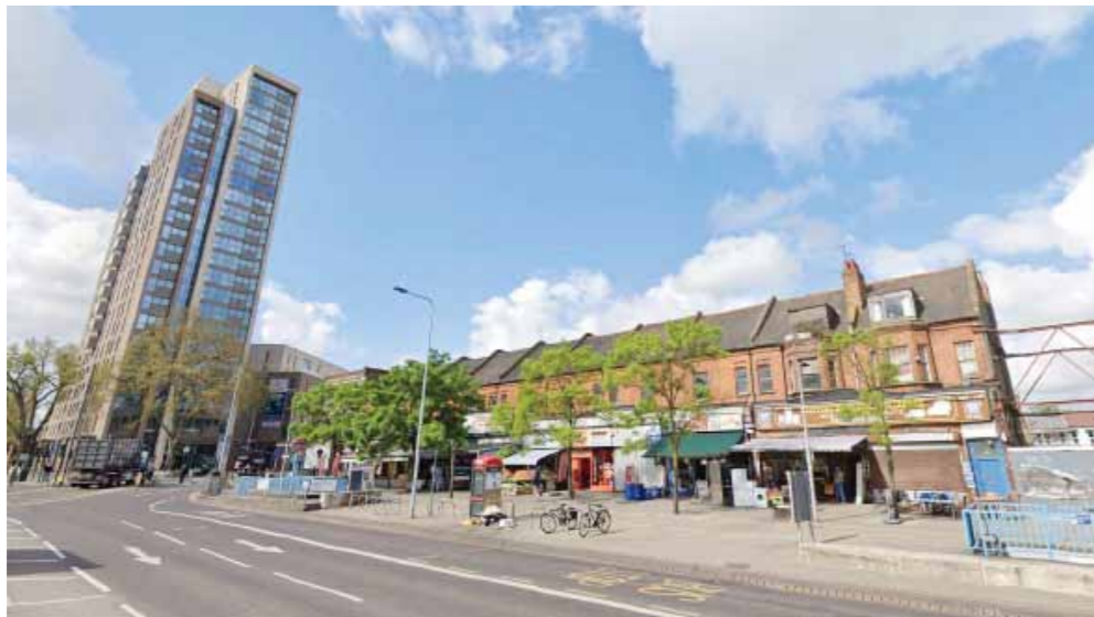
16. Partial view of the wider terrace, 227-249 High Road looking Southward towards the recently constructed 22-storey Apex house Tottenham High Road
