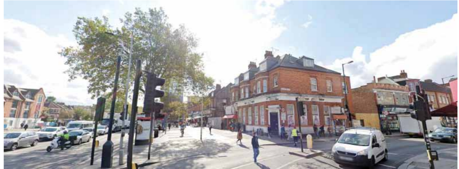
17. View of 259 High Road looking Southward, highlighting the gap in the terrace (the application site) Wood Green Road
